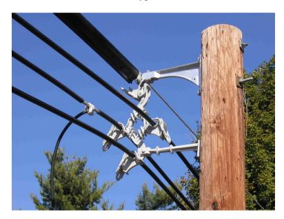
Spacer cable will help prevent outages by hardening the lines. This is a proven technique that we already use and are ready to expand. We will use overhead spacer cable technique in many of these locations and are also looking at targeted undergrounding in specific locations for main line feeders, particularly where ledge is limited, there are few customer interconnections, and there is a heavy tree canopy.
