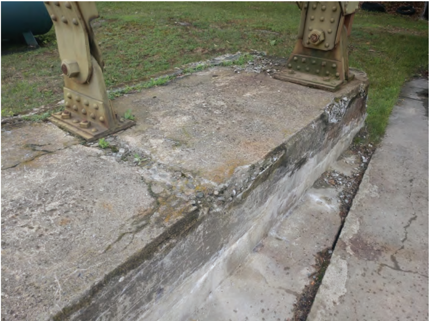
West Bank Foundation
