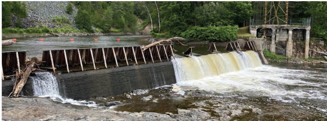
Figure 4-4. Field Photo of the North Spillway Section (Looking Upstream)
