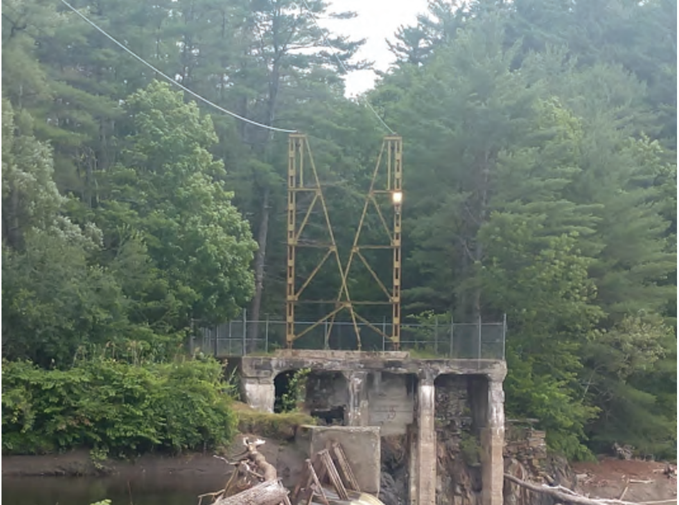
East Bank Foundation and Towers
